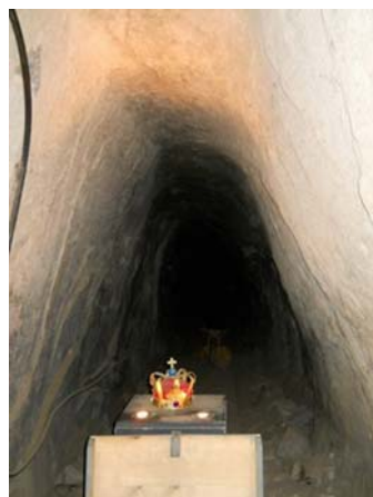
An example of a fireset drift in the Kongens Gruve (King's Mine). Photo by P. Brandes
